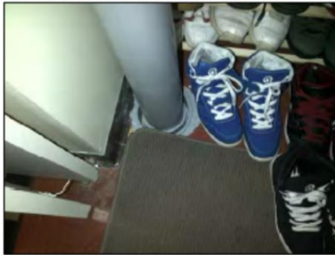
PHOTO 119 - UNIT G3 - SUCTION POINT
